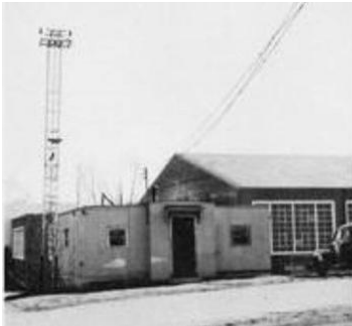
The original WTCC radio station and tower located near the present Memorial Hall.
